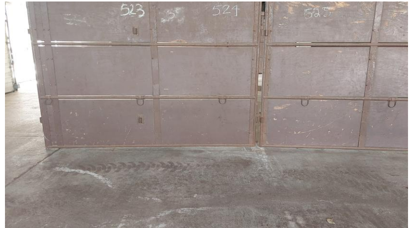
Lower Double Deck Barn Tie Panel
