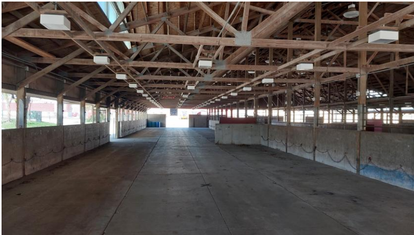
Upper Cattle Barn, Typical Alley
